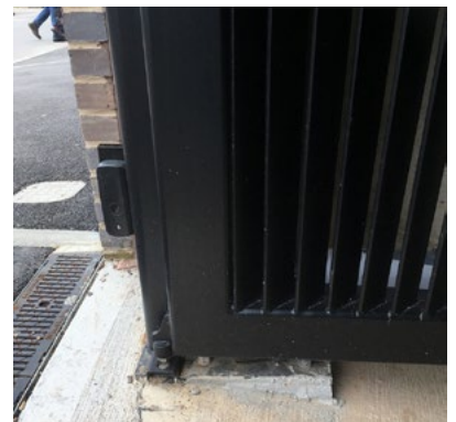
no hinge protection or safety edge where the force is greater nearest the hinge
