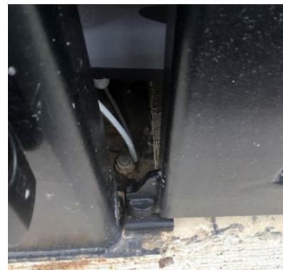
reducing gap and hinge with very high force
