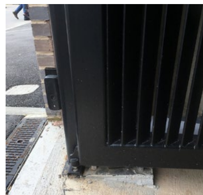
no hinge protection or safety edge where the force is greater nearest the hinge
