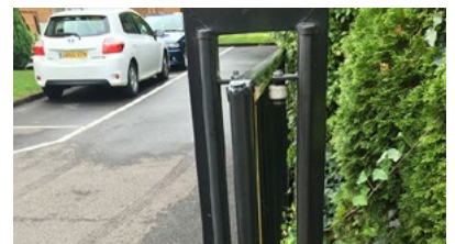
Risk of impact and crushing
