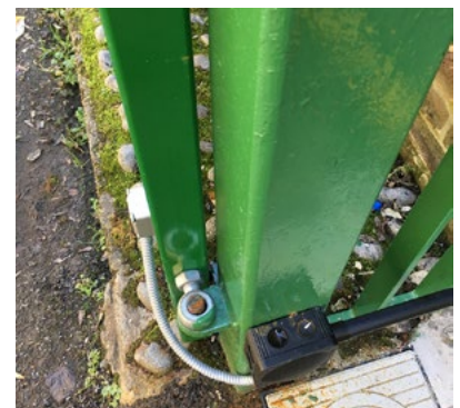
Crushing risk from reducing gap around the hinge
