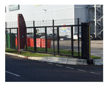
A swing gate using an underground operator clearly has the advantage of not detracting from the aesthetic charm of the gate, however the gate owner would need to be aware of the additional cost associated with installing this type of operator. In addition, maintenance becomes complex due to the limited access. Crank arm operators are typically suited to moving smaller gates. Special attention needs to be paid to the scissor like mechanism to ensure the gate's safe operation.
